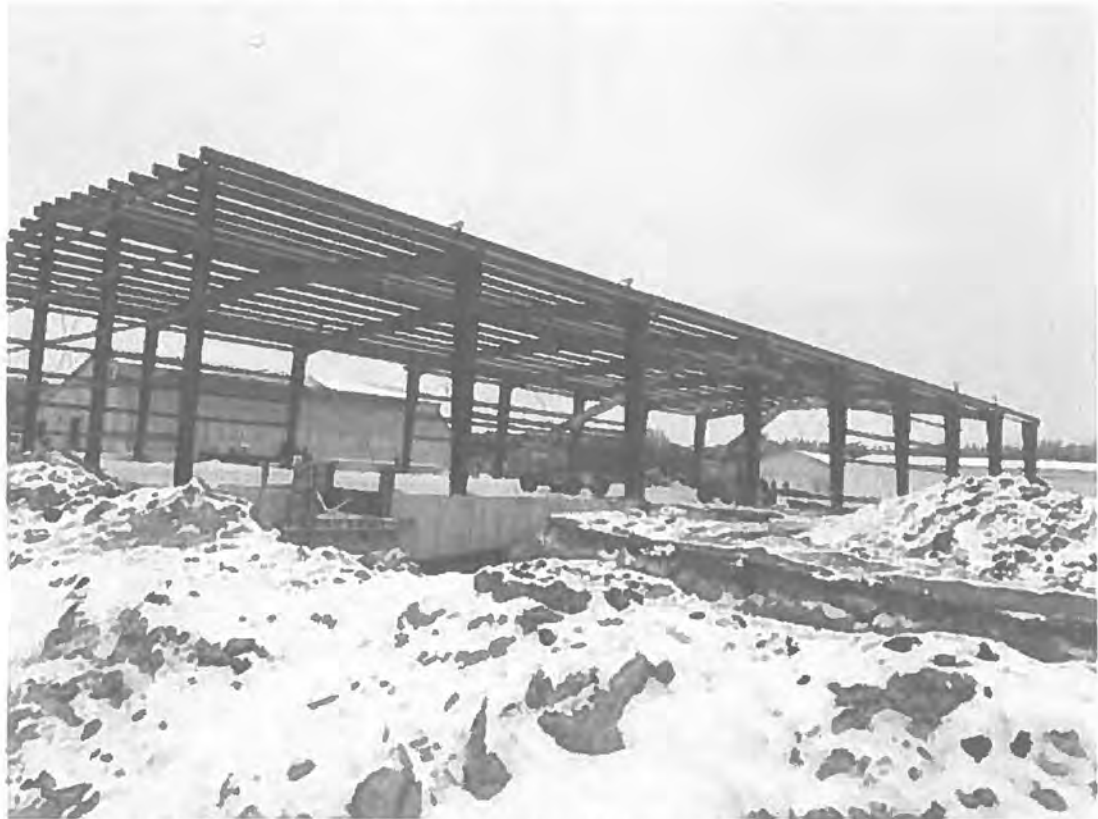
Liquid Fertilizer and Chemical Building Construction as of 12/20/2022
