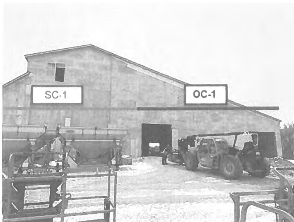
South Side of Dry Fertilizer Building Looking North as of 12/20/2022
